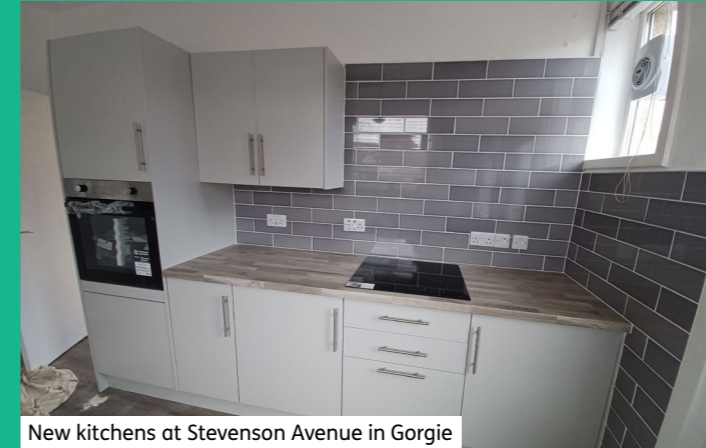
New kitchens at Stevenson Avenue in Gorgie
